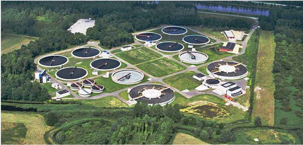
Figure 2.1: Aerial overview of the WWTP Aarle-Rixtel (before installation of fine screens)
